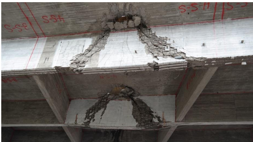
Figure 16 – Photograph of the bridge girders after failure, view from the south (2014-08-26).
